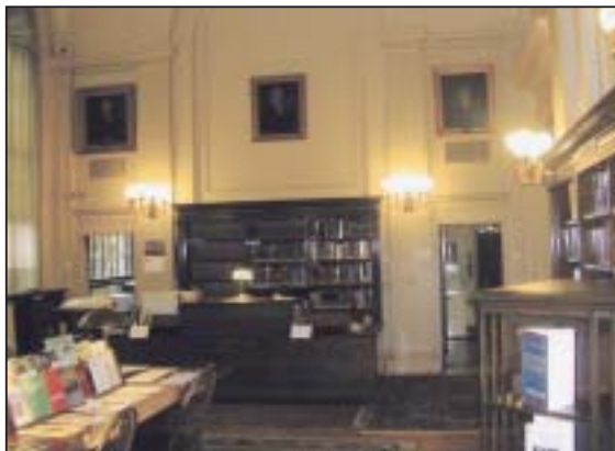
Unobtrusive grilles blend into the décor in the Congregational Library’s historic reading room.
